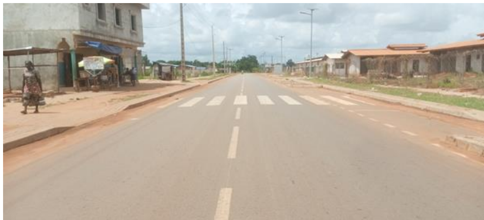
Figure 14. Ouèdo road profile - Residential area under construction
