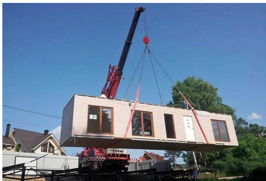
Figure 2. Installation of a large-scale prefabricated volumetric block.
