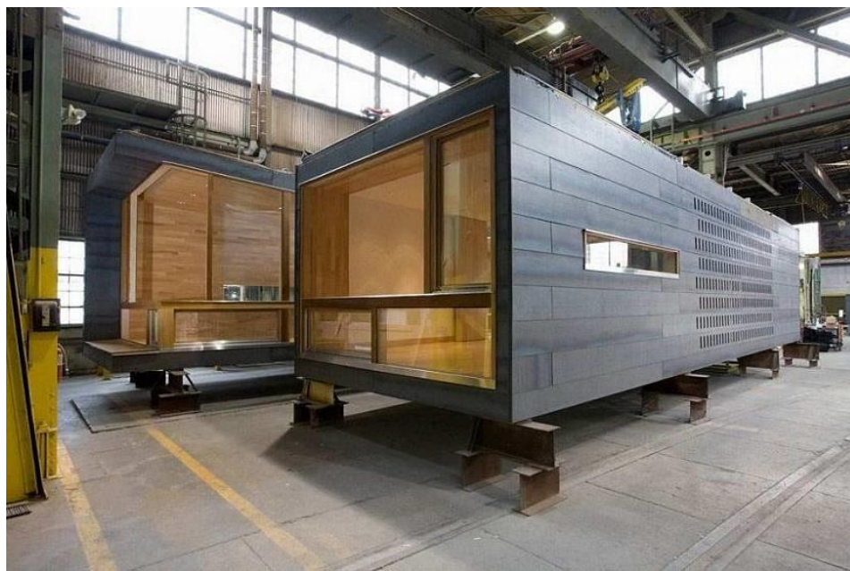
Figure 1. Large-scale volumetric block with advanced prefabrication.
