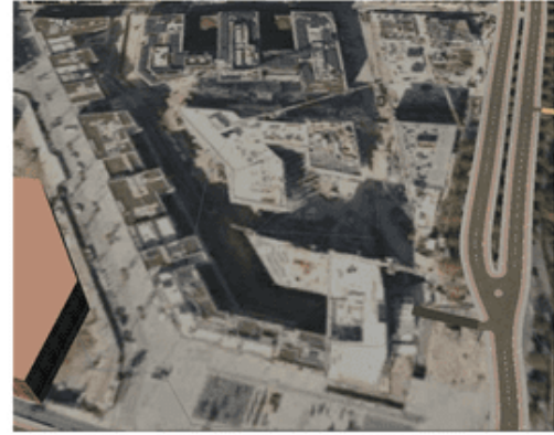
b) Excess buildings removed
