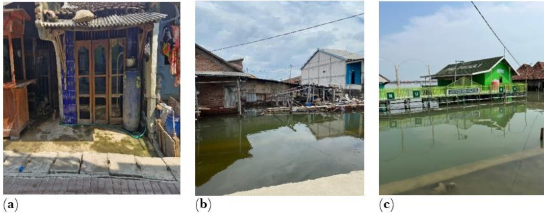
Figure 2. Raising the terrace of the house/building (a); (b); (c).
