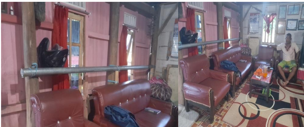
Figure 7. Iron as a support for boards or bamboo if the flood reaches the floor of the house.
