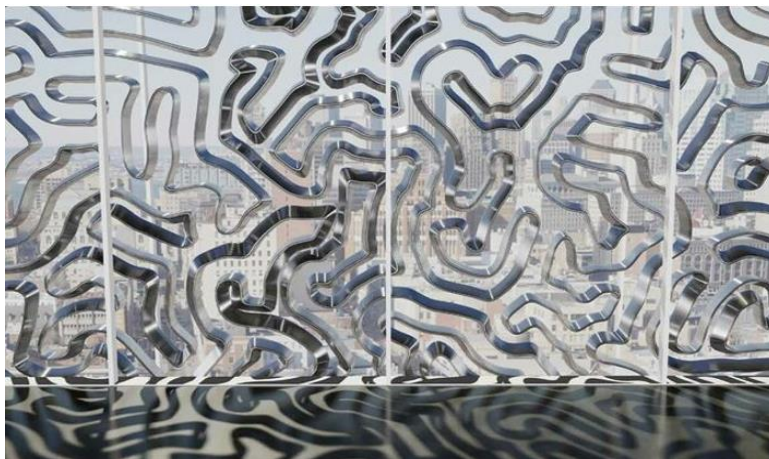
Figure 12. Homeostatic facade system a prototype photo (C)visual simulation courtesy of Decker Yeadon, NY [157].
