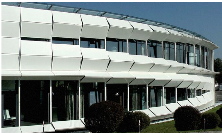
Figure 14. Kiefer Technic Showroom's dynamic facade system [162].
