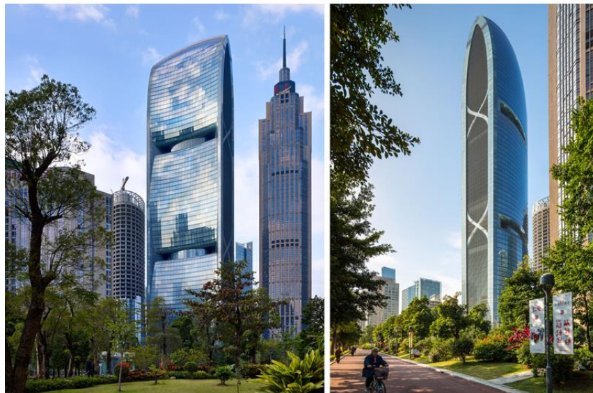
Figure 15. The Pearl River Tower in Guangzhou, China [168, 103].
