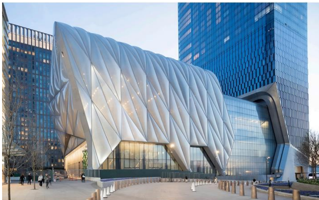
Figure 3. The Shed at Hudson Yards [144].
