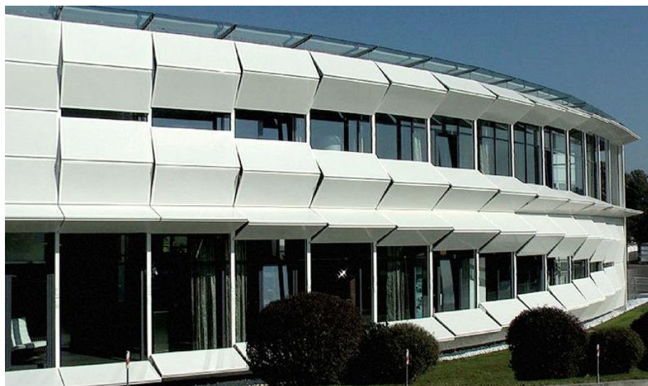
Figure 14. Kiefer Technic Showroom's dynamic facade system [162].
