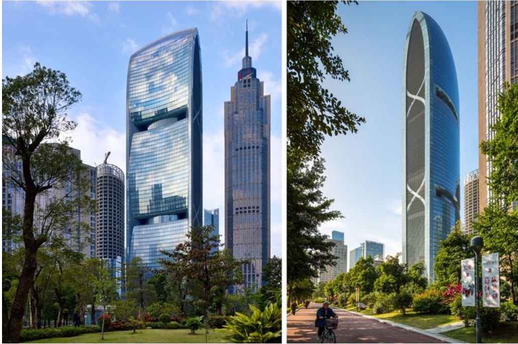
Figure 15. The Pearl River Tower in Guangzhou, China [168, 103].
