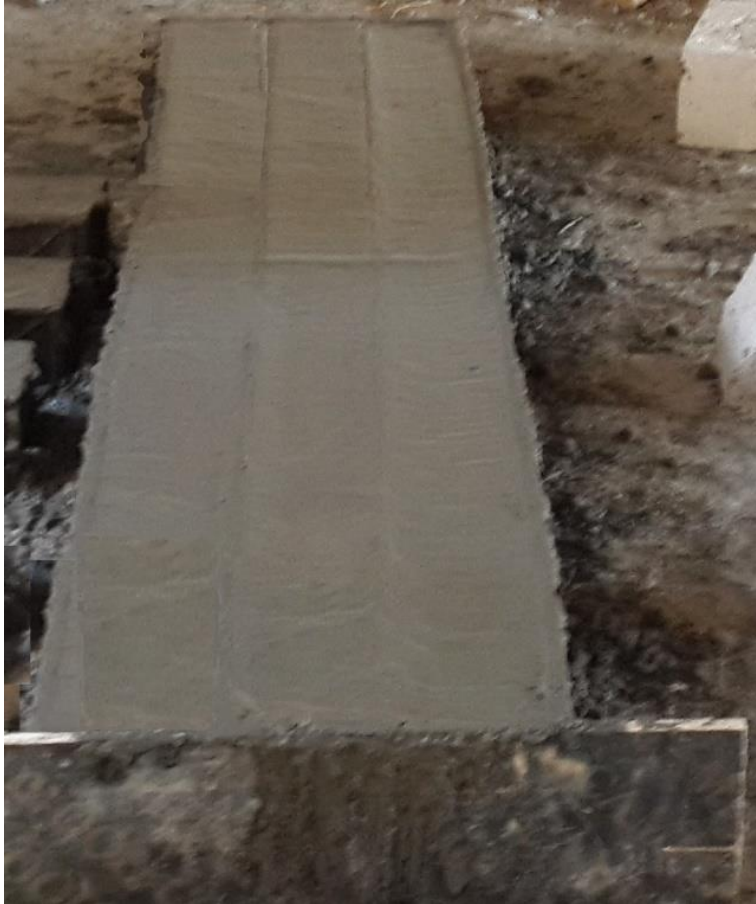
Figure 3. Casting process of reinforced concrete beam samples and their finishes.
