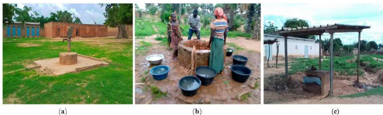
Figure 8. Photo (a) shows a breakdown of a human-powered pump in an elementary school. Photo (b) shows a traditional open-air well used by the local population as a source of water. Lastly, photo (c) shows a non-functional standpipe threatened by water erosion in the town center.
